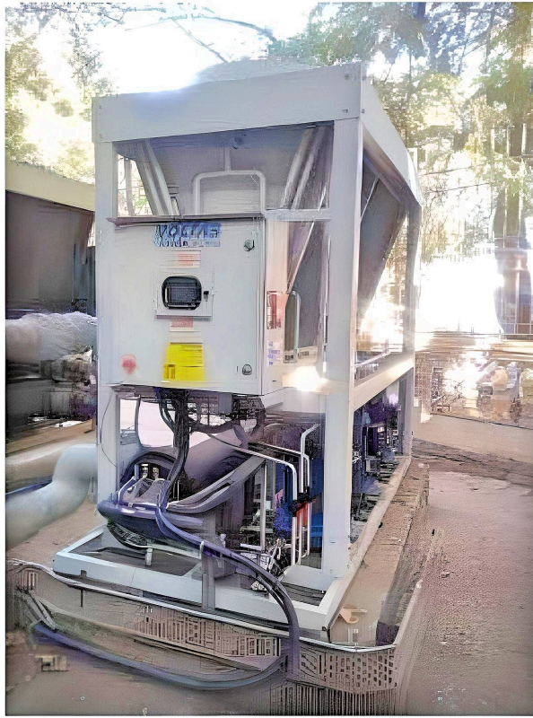
2. Installation of Chiller Plant © CSMVS
